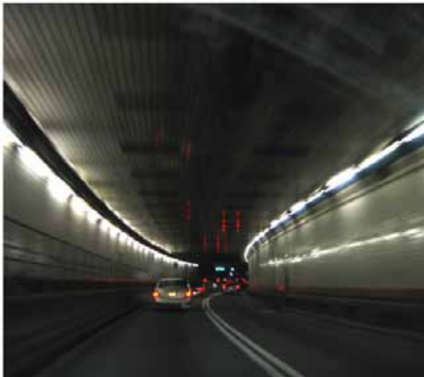
Holland Tunnel en.wikipedia.org
