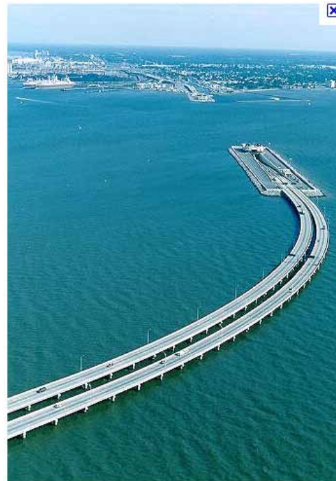
This is a bridge tunnel in Virginia. Notice where it turns into a tunnel to go through the water. Photo by Virginia Department of Transportation.
