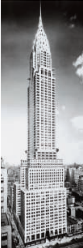
15-B.1 William Van Alen (1883–1954), The Chrysler Building, Manhattan, 1926–1930 (photographed in 1930). Located at 42nd Street and Lexington Avenue, New York. Steel frame, brick, concrete, masonry, and metal cladding, height 1046 ft. (318.82 m.). Photographic print. Library of Congress, Prints and Photographs Division, Washington, D.C.
